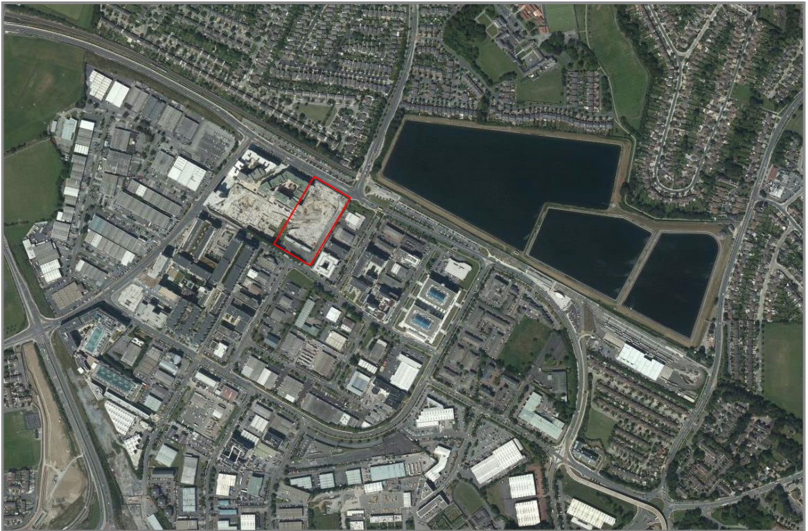
Figure 10.4: Aerial Image of Site.
